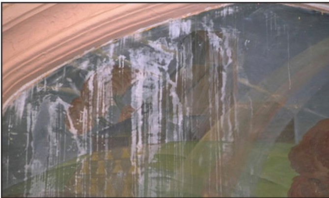
Fig. 7: Evidence of water damage.
