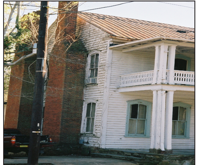
Fig. 7: Detail of chimneys, deteriorated wood siding and metal roof of the Colonial Inn.
