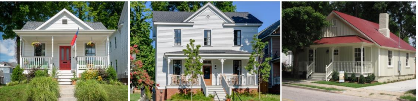
Shaffer House, Raleigh; Gorham House (now Guest House Raleigh), Raleigh; 811 S. East Street, Raleigh
