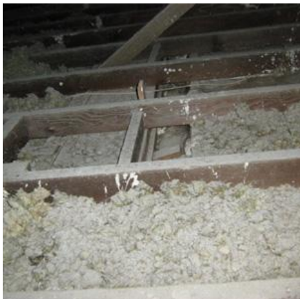
Blown in Attic Insulation
