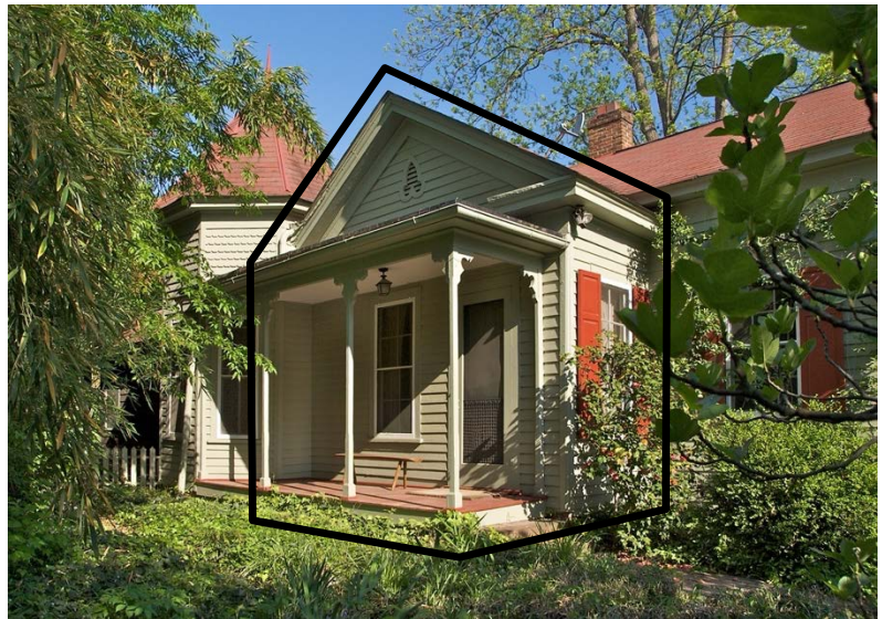
This portion of the building dates from the original 1869 construction.
