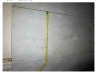
In contrast to the plainer finish of many log houses, the care devoted to building the King House appears in such hallmarks of "neat and workmanlike" craftsmanship as the beaded ceiling joists, heart pine floors, batten doors hung with hand-wrought HL hinges, and beaded tongue-and-groove sheathing of the walls, made of hand-hewn boards over 20 inches wide, which recall the massive trees of the old forests in the area.
